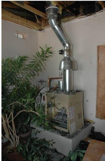
**Figure 3 – The floor heating system boiler in the garage of the residence. The capped gas line protruding from the wall and the nearby water heater and furnace closet can be seen behind the boiler.**
