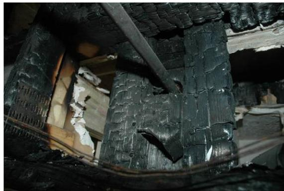
**Figure 6 – The area where the gas line entered the end of the insulation-filled wall cavity.**
