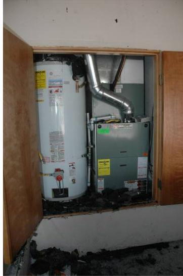
**Figure 4 –The water heater and furnace closet. Note the lack of fire damage in the closet.**
