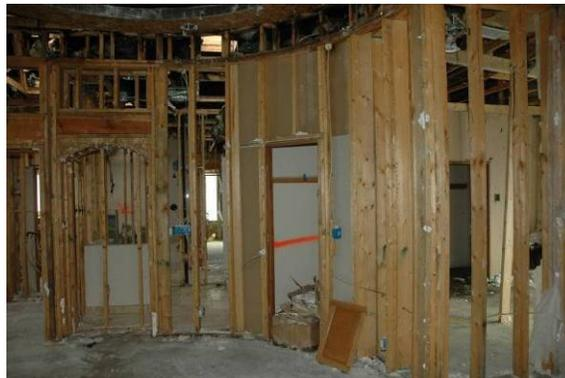
**Figure 2 –The residence interior after the fire and after the sheetrock had been removed.**
